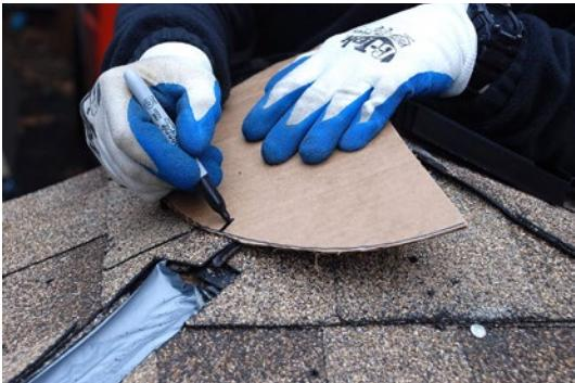
**STEP 7 —** Rotate the template around to the front roof plane. Align the first angle to right hip. Mark a second angle on the template for the left hip. Use a straight edge to draw a line connecting the second mark to the template notch.
