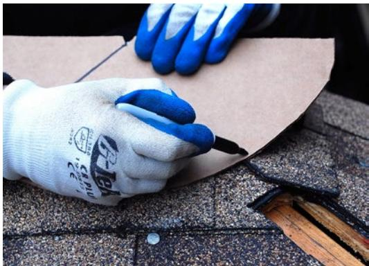
**STEP 3** — Align the template to the **top right corner** of the Cobra® Hip Vent and mark the two angles on the top of the vent.
