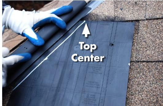
**STEP 10 —** Snugly fit Cobra® Hip Vents together and with the ridge vent. Fasten the hip vents into place using 1 3/4" (44 mm) coil nails through the pre-marked 6" (152 mm) increment nail gun targets. Use a 3" (76 mm) wide strip of WeatherWatch® or StormGuard® Self-adhering Leak Barrier to cover any joints between vents.
