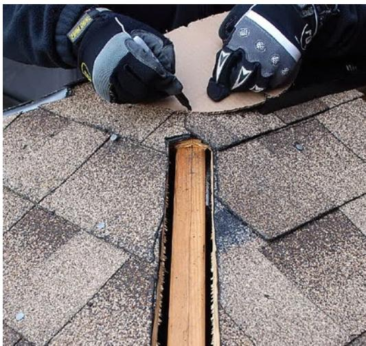
**STEP 2** — Rotate the template around to the front roof plane. Align the first angle to the left hip. Mark a second angle on template for the right hip. Use a straight edge to draw a line connecting the second mark to the template notch.
