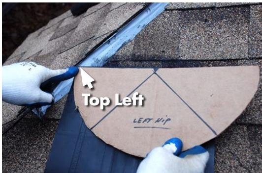
**STEP 9 —** Locate the top center of the Cobra® Hip Vent. Use a straight edge to draw two lines from the **top center** through the two previously marked angles. Carefully cut the vent along the two lines as shown in **Step 5**. The left hip vent section is now complete.
