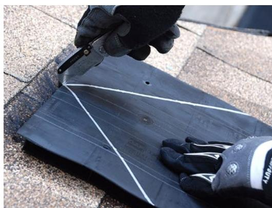
**STEP 6 —** Flip the template over and use it to find the angles for the left hip. Mark the first angle for the left hip on the template. Use a straight edge to draw a line connecting the mark to the **template notch**.
