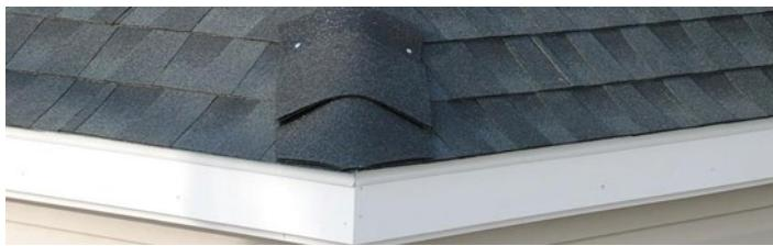
**Starting at the bottom of the hip nearest the eave:** Center and conform Cobra® Hip Vent over the shingles, placing it firmly against the roof surface.
