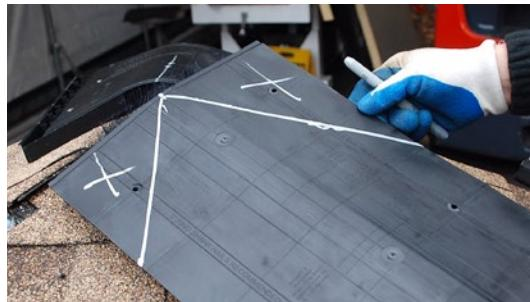
**STEP 5** — Carefully cut the Cobra® Hip Vent along the two lines. The right hip vent section is now complete.
