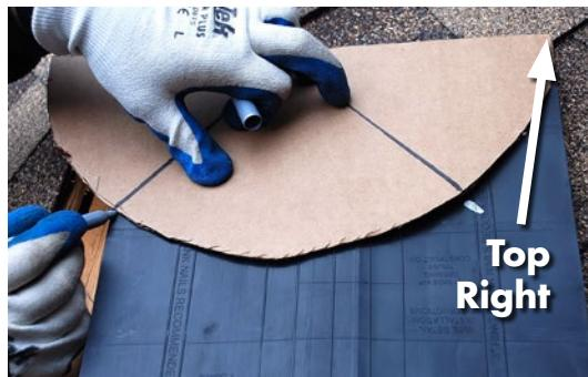
**Note:** The "Towards Peak" arrows embossed on the top surface of the vent should always point towards the peak of the roof.
