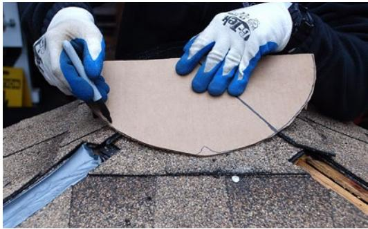
**STEP 8 —** Align the template to the **top left corner** of the Cobra® Hip Vent this time, and mark the two angles on the top of the vent.
